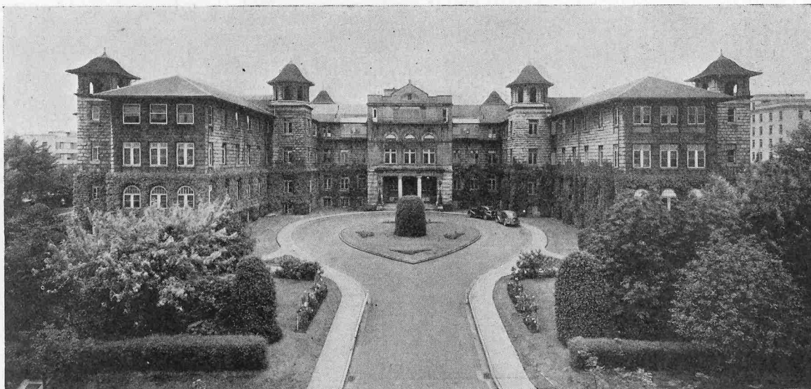
Fig. 7—Present appearance of the Main Building of the Vancouver General Hospital.
